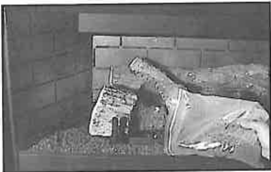
Figure 46 - Placing Lava Rock
