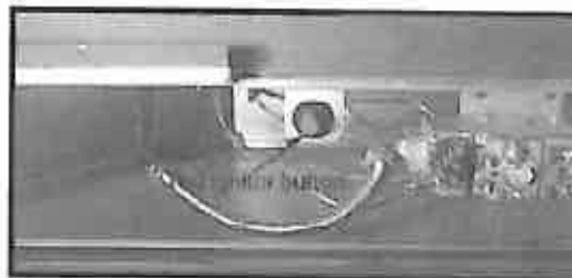
Figure 50 Typical Standing Pilot Ignition
