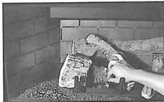
Figure 48 - Placing the Rock Wool
