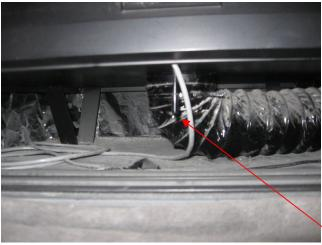
Above is the vinyl duct & the lever that appears to open & close some type of damper. The wire that you see is from a previous remote control for the gas logs.
