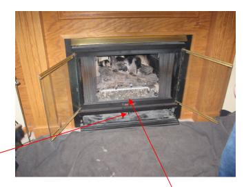
This is the front view. If you look close you can see the "damper" lever. I can feel with my fingers a "channel" in the front of the firebox where I assume it allows air to enter the firebox from the bottom.
