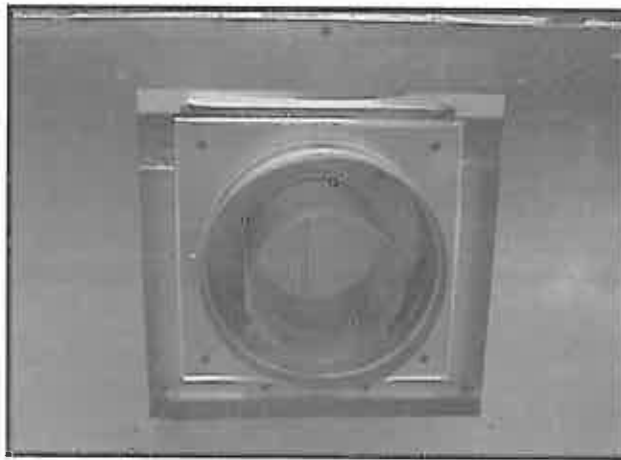
Figure 14 - Place Outer Collar on Rear of Appliance
