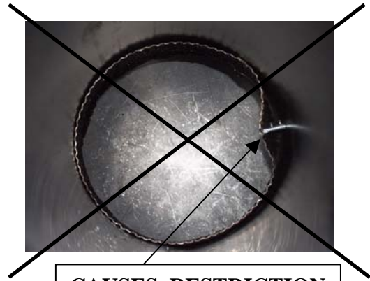
FAULTY INSTALLATION
