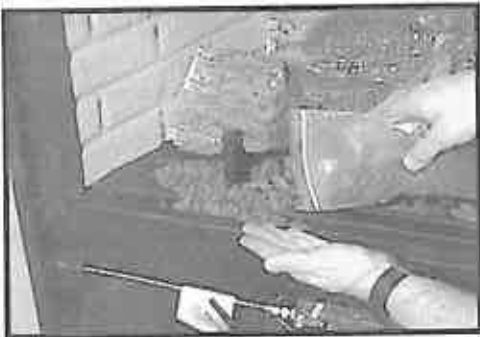
Figure 46 - Placing the Lava Rock
