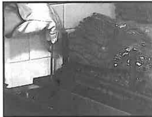
Figure 36 Unscrewing the Log/Grate Assembly from the Hearth Pan
