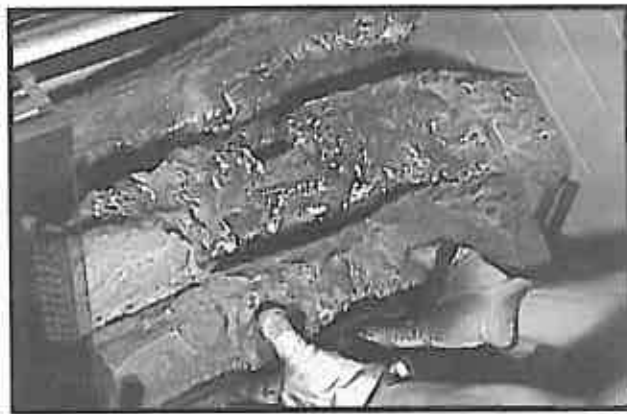
Figure 25 Log Removal
