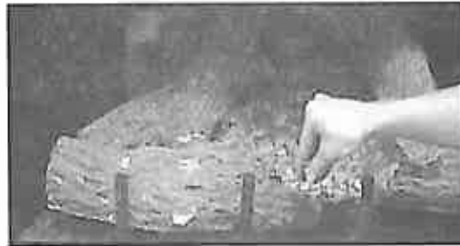
Figure 21 - Placing the Vermiculite
