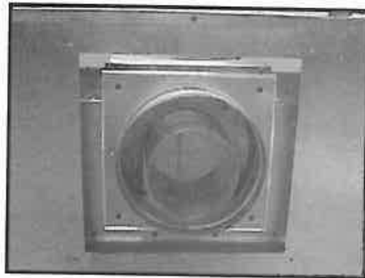
Figure 14 - Place Outer Collar on Rear of Appliance
