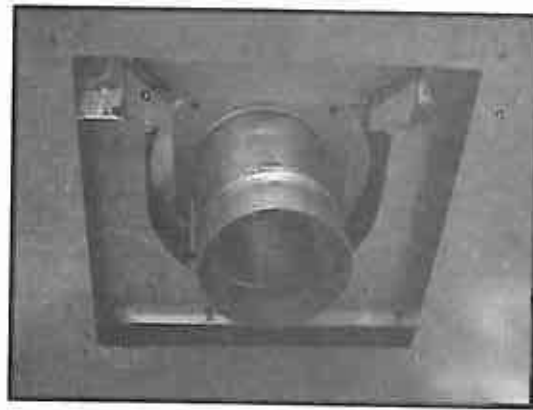
Figure 13 - Place Inner Collar on Rear of Appliance
