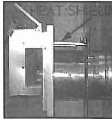
Figure 26 Vent Wall Shield and Termination Cap
