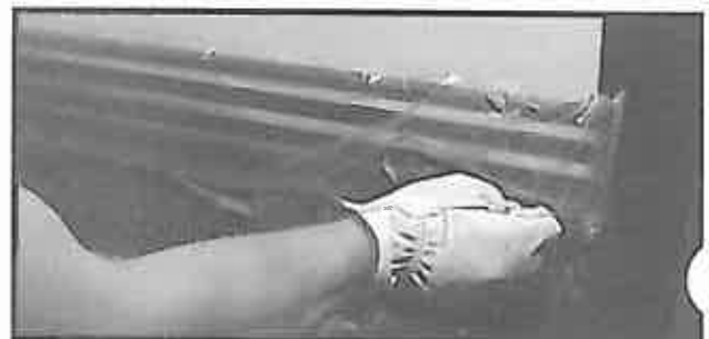
Figure 21 - Control Access Panel Removal
