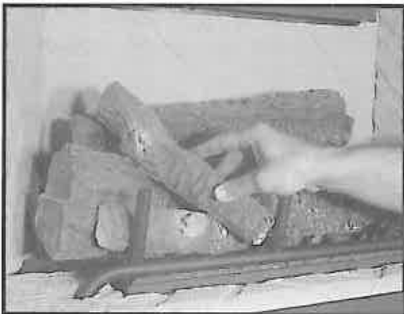
Figure 61 - Placing Top Left Log (Natural Gas Shown)
