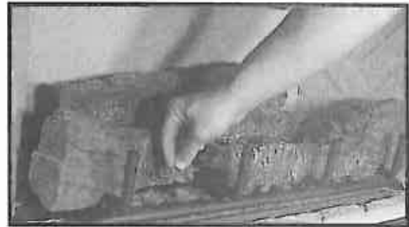
Figure 56 - Placing the Rock Wool
