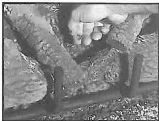
Figure 20 Placing the Fire Glow
