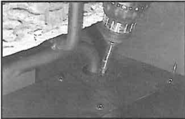
Figure 32 Unscrewing the Log/Grate Assembly from the Hearth Pan
