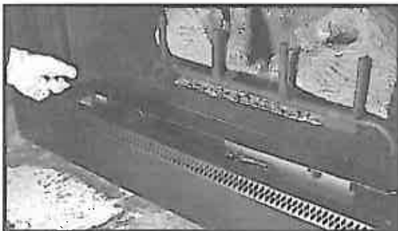
Figure 11 - Control Access Panel Removal
