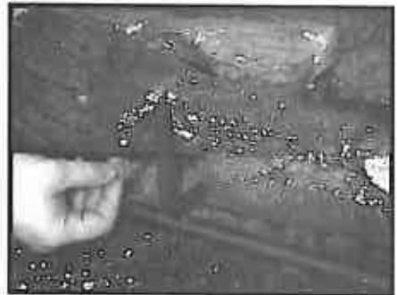
Figure 29 - Placing the Rock Wool
