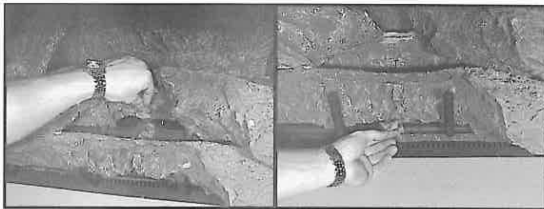
Figure 17 Placing the Rock Wool
