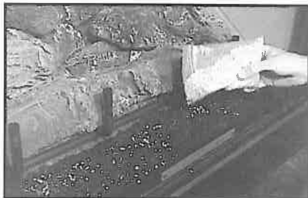
Figure 16 Placing the Vermiculite
