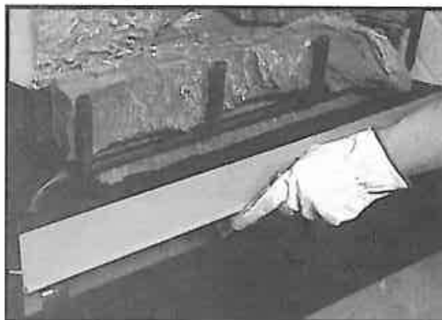
Figure 11 Control Access Panel Installation/Removal
