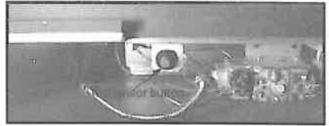
Figure 50 Typical Standing Pilot Ignition
