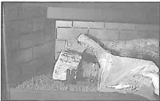
Figure 46 - Placing Lava Rock
