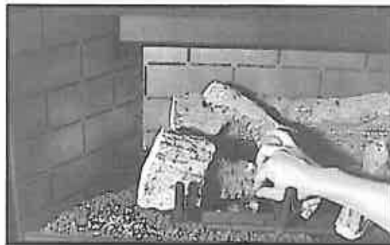
Figure 48 - Placing the Rock Wool
