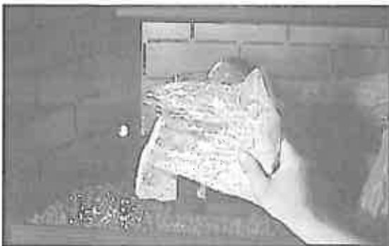
Figure 47 - Placing the Vermiculite
