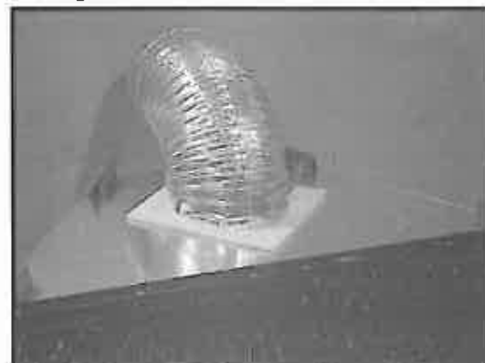
Figure 9 - Attach the First Vent Section
