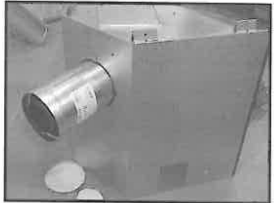
Figure 12 - Attach the First Vent Section
