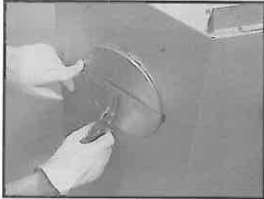
Figure 10 - Cut the Retaining Band
