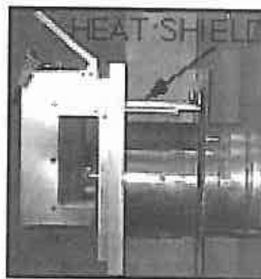
Figure 22 Vent Heat Shield and Termination Cap
